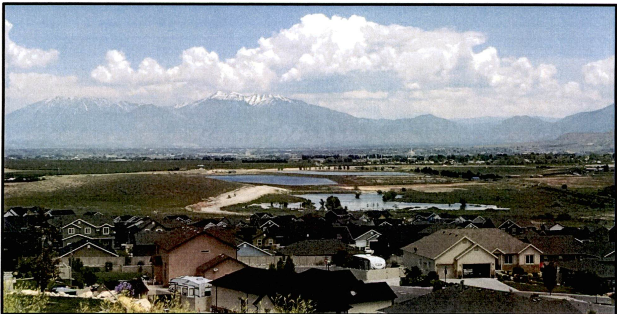
Extension of Summit Ridge Parkway to US-6 Main Street Under Construction – June 2019
