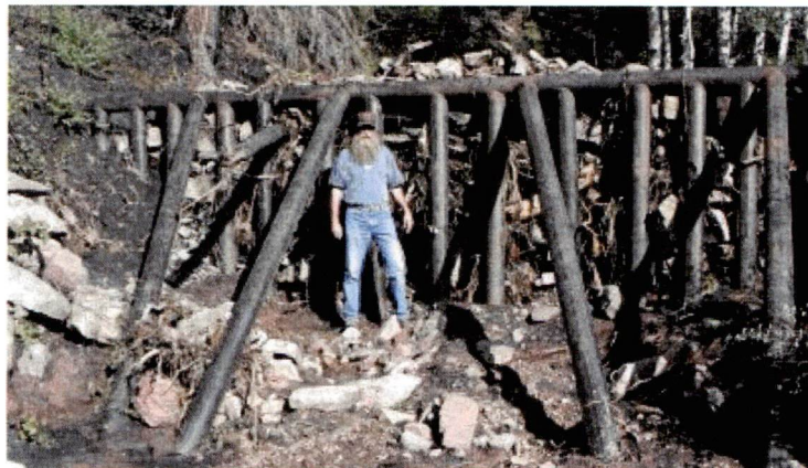
Figure 5. Debris rack installed near Lemon Dam, CO.
