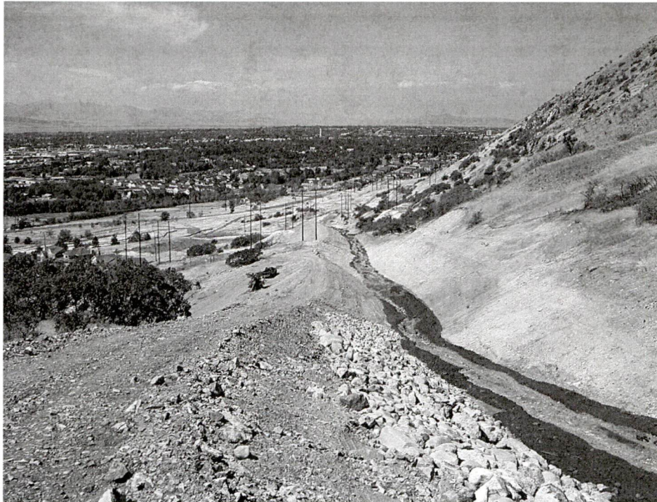
Figure 8. Downstream view of the Buckley Draw deflection berm near Provo, Utah, after a small debris flow (from Elliot, 2007).
