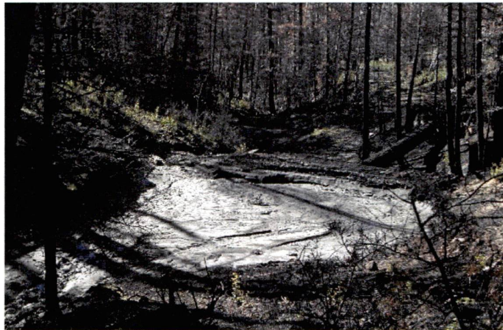
Figure 7. Check dam that captured ash/mud runoff following a rainstorm near Lemon Dam, CO.
