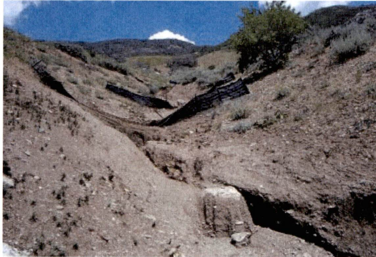
Figure 4. Failed silt fences near Farmington, UT.
