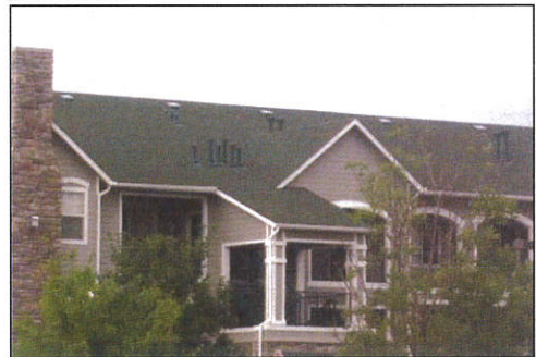
Appropriate roof top equipment treatments
