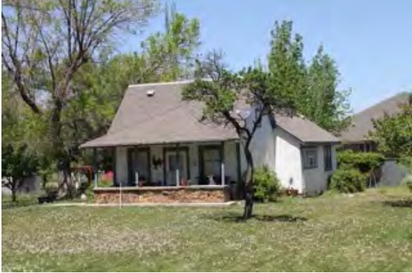
Hall and Parlor 369 E 100 N
