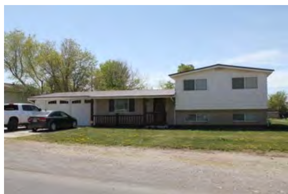
Split Level 158 S 100 E
