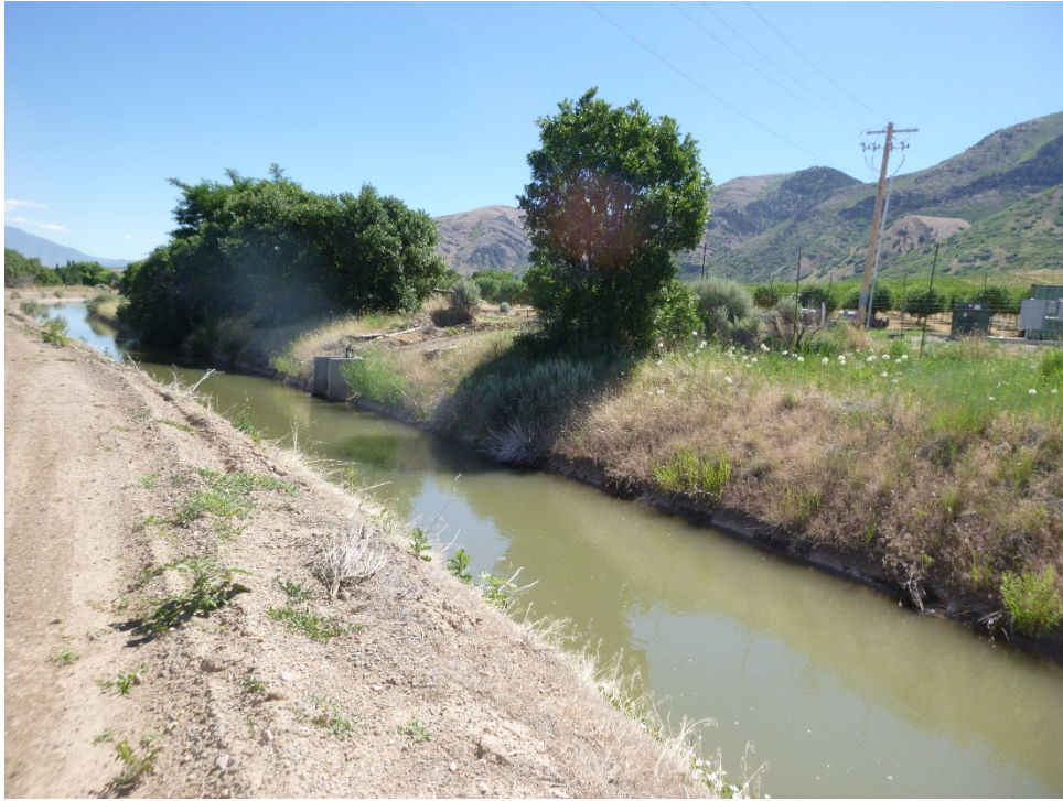
Figure 3- Strawberry Highline Canal looking northeast
