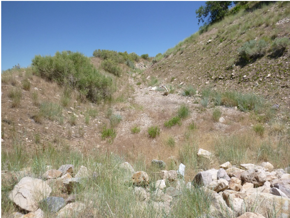
Figure 6- Depression near outflow location 4
