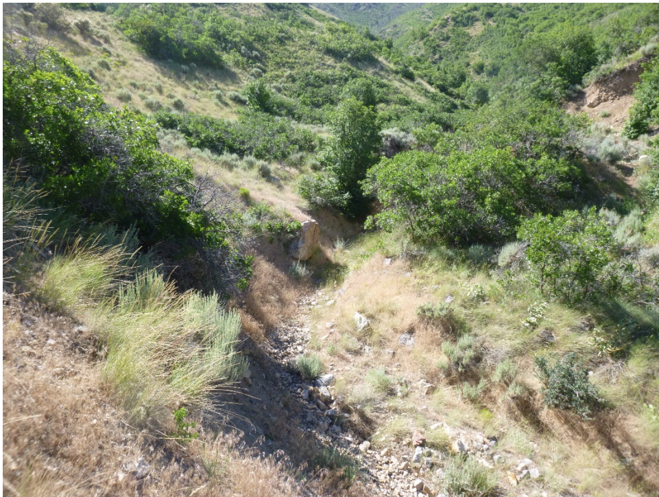
Figure 1- Depression near outflow location 6
