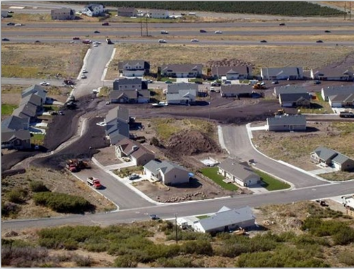
VIEW OF DAMAGE CAUSED BY DEBRIS FLOW 2002
