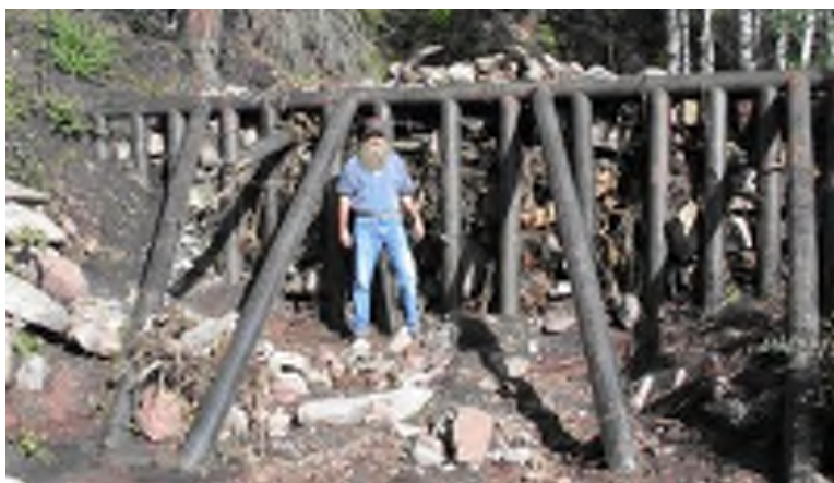
Figure 5. Debris rack installed near Lemon Dam, CO.
