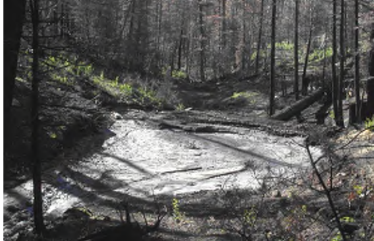
Figure 7. Check dam that captured ash/mud runoff following a rainstorm near Lemon Dam, CO.
