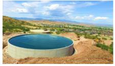
Last year, we completed a major initiative to install a new 3-million-gallon pressurized irrigation water tank and booster pump station on our east bench. The vast majority of our east bench residents are now using water from an irrigation water sources that is feeding our irrigation water system. This project dramatically reduced the draw from our culinary water system and improved the overall operations of both systems.
