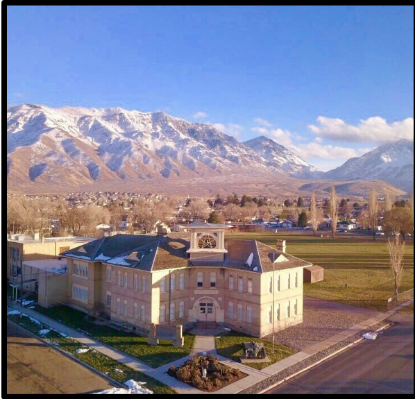
Old Rock School House Corner of 100 South and 100 West
