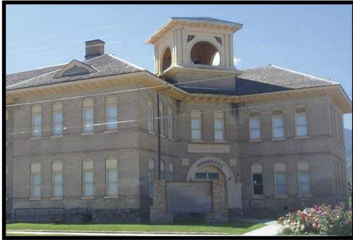
Old Rock School House Corner of 100 South and 100 West
