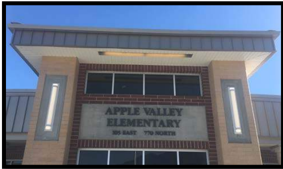
Newly Constructed Apple Valley Elementary School opens August, 2018
