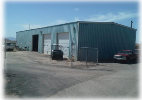
Old Public Works Building built in 1972
